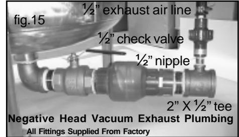
An alternative is to pipe the vacuum exhaust to a location where the odor does not bother anyone.
